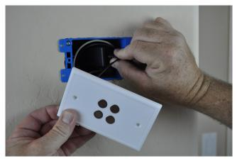
3. Using the supplied #2 Philips head screws, mount the plate. Make sure the S-Mount is tight to the wall. Do not overtighten and bend the S-mount, the face should remain flat.
