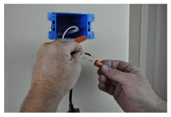
2. Carefully place the power supply into the electrical box as far as possible, it will need to be at least 1/2" in from the face of the electrical box for the S-Mount to fit.
