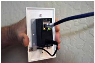
5. Using the supplied #2 Philips head screws, mount the plate. Make sure the S-Mount is tight to the wall. Do not overtighten and bend the S-mount, the surface should remain flat with the screws flush with the face.
