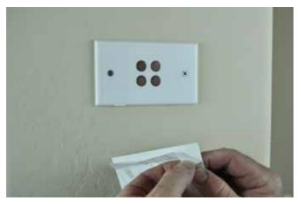
7. Starting at one corner, align the long edge of the rubber face to the indent on the S-Mount. Adjust as necessary. Once the alignment is perfect, then press the edge onto the S-Mount.
