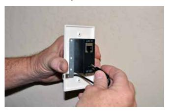
4. Plug the Cat5/Cat6 cable that runs from the injector into the rear of the S-Mount-POE. If the connection is good, both LED's will light.
